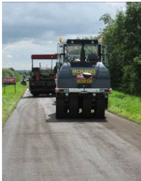
Cold emulsion 100% recycled asphalt surface course
