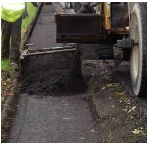
Cold emulsion structural asphalt installation and core specimen.
