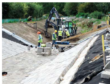
↑ Channel restoration works in progress SHROPSHIRE UNION CANAL SOCIETY
