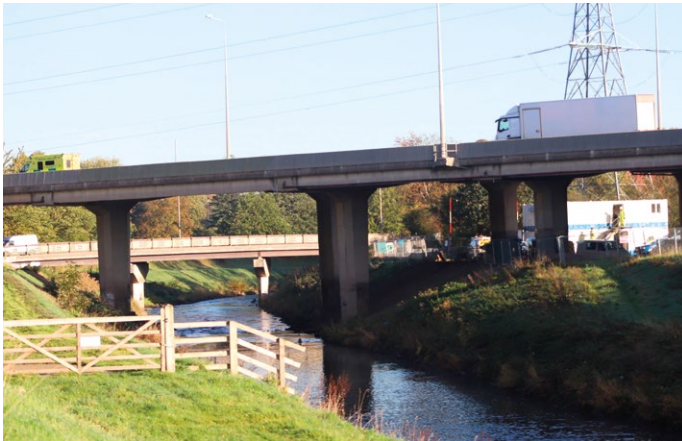
↑ Repair work beneath the M60 bridge over the River Mersey involves the use of temporary supports and hydraulic jacks (right) HIGHWAYS ENGLAND
