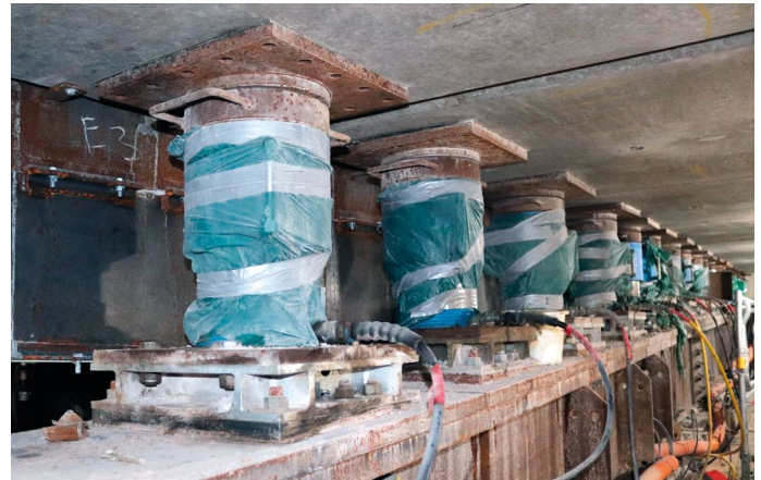
↑ Repair work beneath the M60 bridge over the River Mersey involves the use of temporary supports and hydraulic jacks (right) HIGHWAYS ENGLAND
