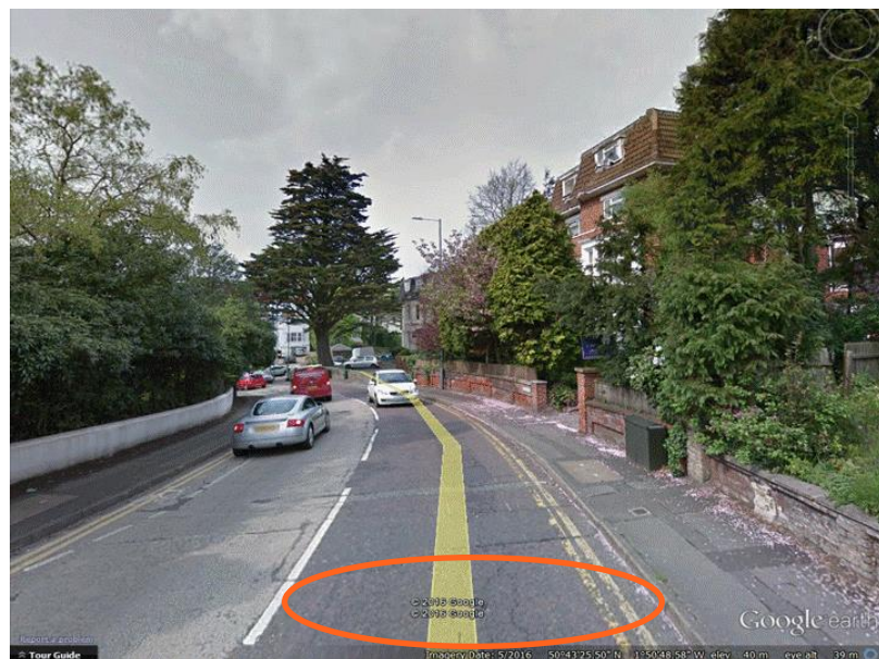
Figure 74: Sunken trench on Boscombe Road reported to contain a bump in 2013 and 2015
