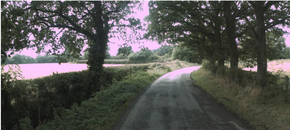
Figure 16: The forward facing image of fretting, seen on the SRR2 extension route
