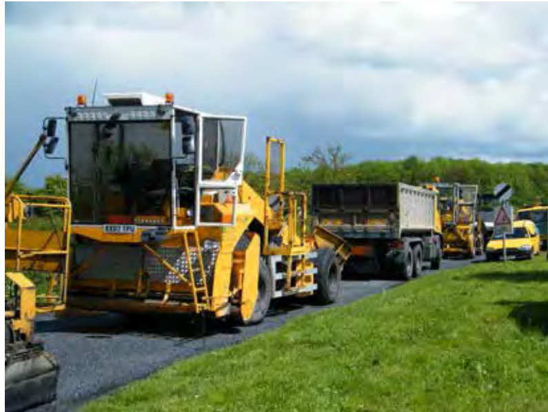
Planned Maintenance at Leicestershire County Council
