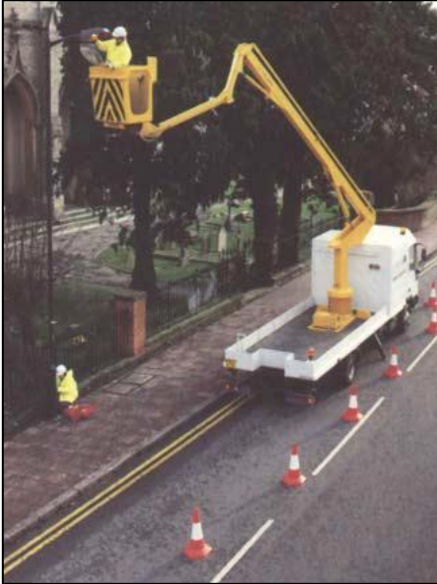
Figure 4.1: Maintenance of 8 m lighting unit. Photograph reproduced by permission of Parkersell Highway Lighting Ltd.
