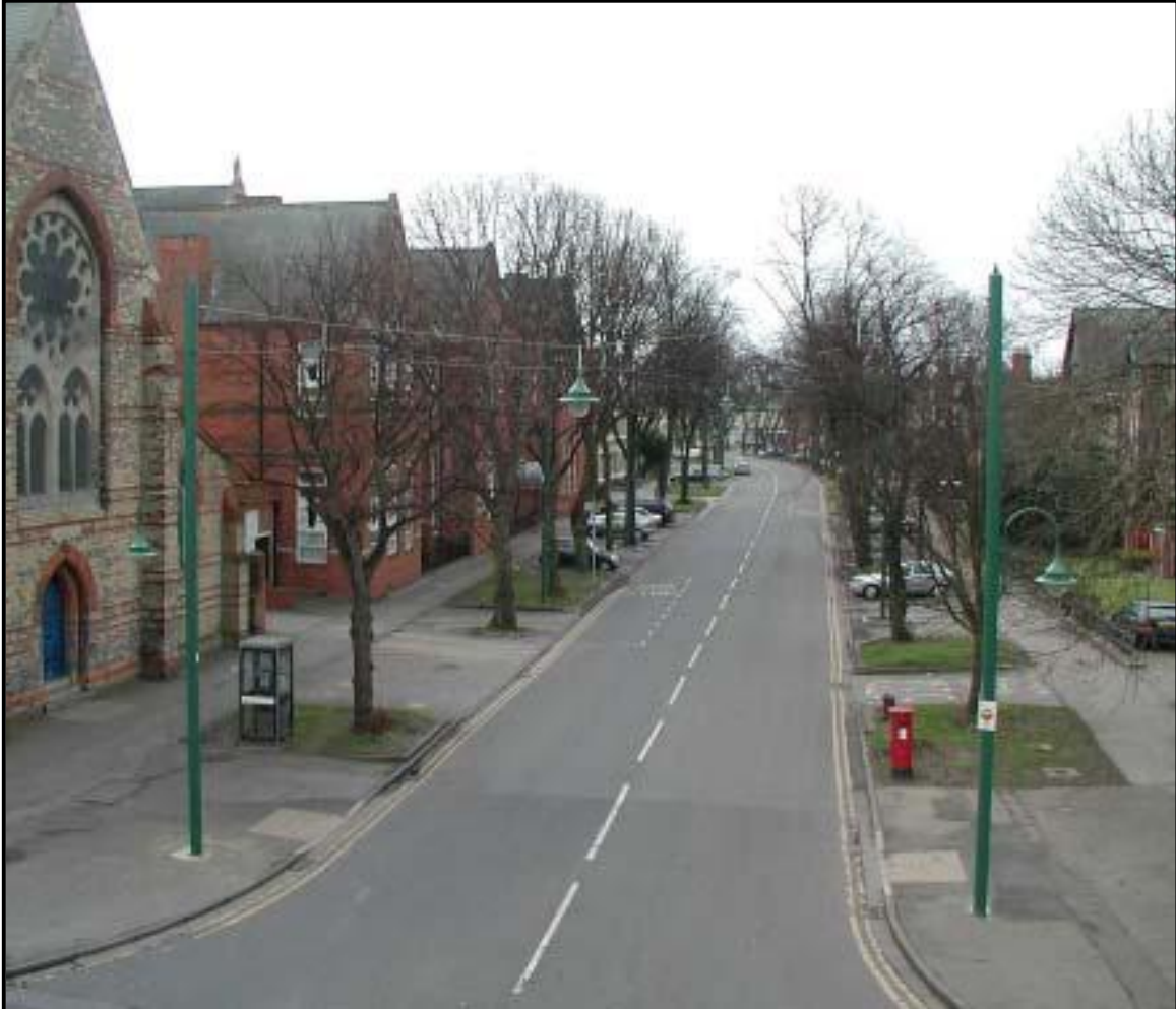
Figure 3.1: The Boulevard, Kingston upon Hull. A lighting scheme designed to light a heavily treed boulevard without extensive pruning of the trees. The carriageway lighting is provided by centrally mounted catenary suspended luminaires using high pressure sodium lamps. The footway lighting is provided by secondary luminaires mounted on the rear of the lighting columns using ceramic metal halide lamps. Photograph by kind permission of Sugg Lighting Ltd.
