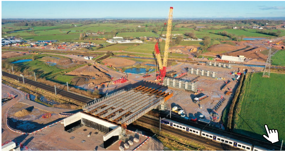
↑ Beams for a new viaduct were installed over a railway line in Lancashire
