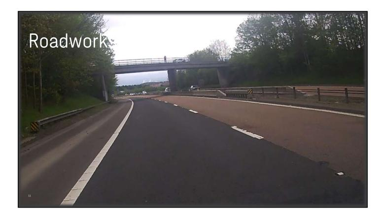
Roadworks often see permanent infrastructure being removed to be replaced or upgraded. In this situation the central reservation barrier is being replaced overnight, with higher containment being provided at the bridge pier. However, the temporary barrier is not rated for the national speed limit motorway, which is reopened to two lanes and hard shoulder for daytime traffic.
