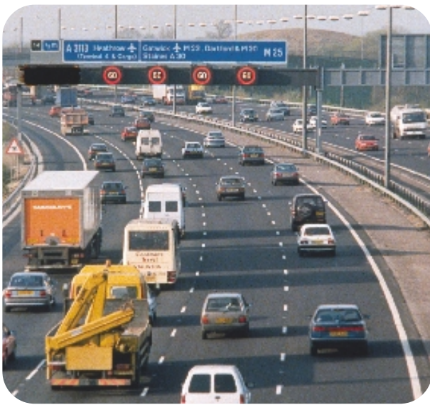
Speed-controlled motorway (M25). (Highways Agency).
