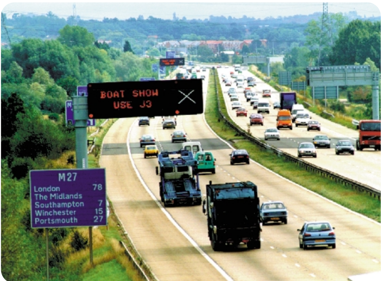
Use of VMS for strategic re-routing. (Highways Agency).
