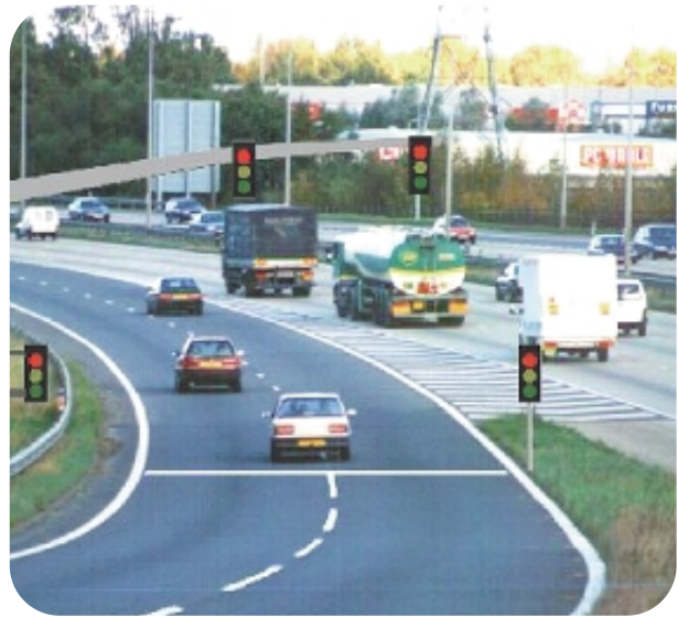
Ramp meters control access to the motorway. (Highways Agency).
