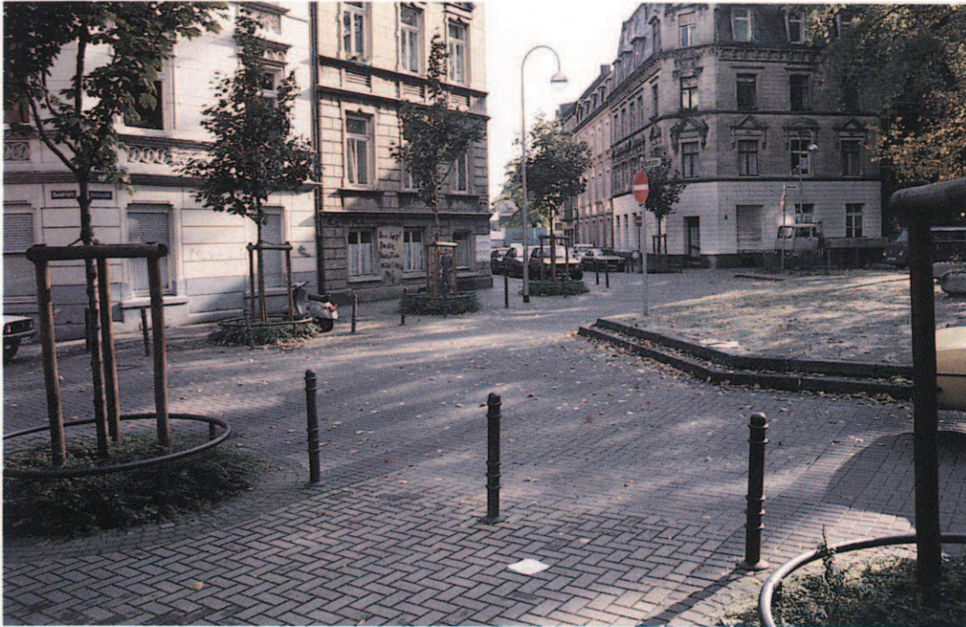
18: Paving details in the Nippes district now reflect the geometry of buildings rather than the geometry of traffic. Here part of the street has been raised, forming a "stage" at the entrance to a church. (Photo: T. Pharoah)
