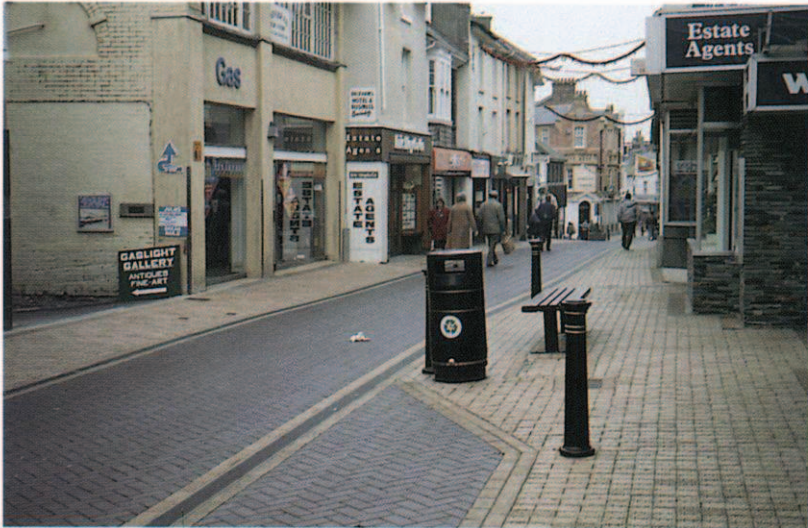
64: Carriageway and footways paved at one level. Contrasting colours define the vehicle track. (Photo: Devon County Council)
