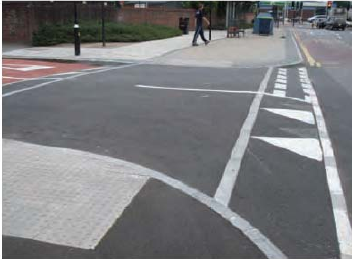
At Grade Crossing Point
