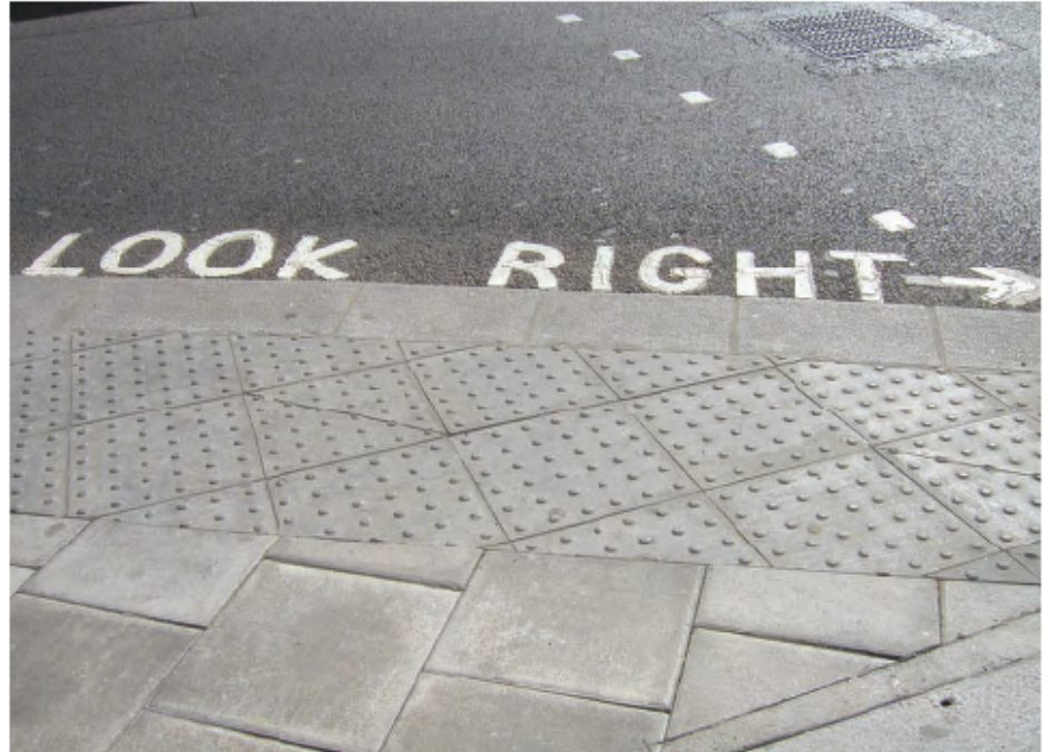
Grey concrete blister tactile paving laid in line with the angle of the crossing, in accordance with DETR guidance
