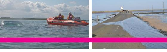
The choice of limiting the road height above sand level to 9 inches (225mm) has proved very foresighted. On occasions when resurfacing schemes have raised the road above that level, a winter storm restores the status quo. The sea rolls the additional road surface up just like a carpet and deposits it to the carriageway edge. In recent years edge restraints to the carriageway have formed part of resurfacing schemes.
