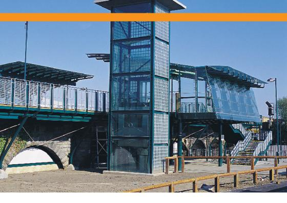
At Fellgate Station, lift shafts were built without disturbing the 160-year-old railway embankment on the route of the original 1839 Brandling Junction Railway. St Peter's Station, north of the River Wear, was built without damaging the listed stone viaduct it sat upon. The challenge led to construction of an eye-catching glass building which has become one of the icons of the whole line.
