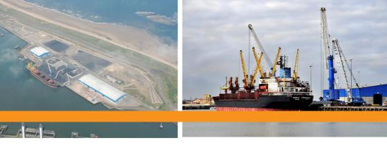
Alcan Bulk Terminal is a deep water (10.4m) import terminal which handled 0.5 million tonnes per year of Alcan raw materials, until the aluminium smelter closed in 2012. It has a rail link and storage silos.
