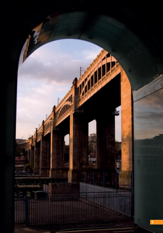
The High Level Bridge has six river spans of 125 feet (38m) length, sitting on masonry piers 46 by 16 feet (14 by 4.9m) in section and up to 131 feet (40m) height. There are also four land spans on each side, of 36 feet 3 inches (11m). The single carriageway road and pedestrian walkways occupy the lower deck of the spans, 85 feet (26m) above the high water mark, and the railway the upper deck 112 feet (34m) above the high water mark. The total weight of the structure is 5,000 tons.
