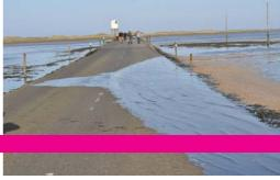
The choice of limiting the road height above sand level to 9 inches (225mm) has proved very foresighted. On occasions when resurfacing schemes have raised the road above that level, a winter storm restores the status quo. The sea rolls the additional road surface up just like a carpet and deposits it to the carriageway edge. In recent years edge restraints to the carriageway have formed part of resurfacing schemes.
