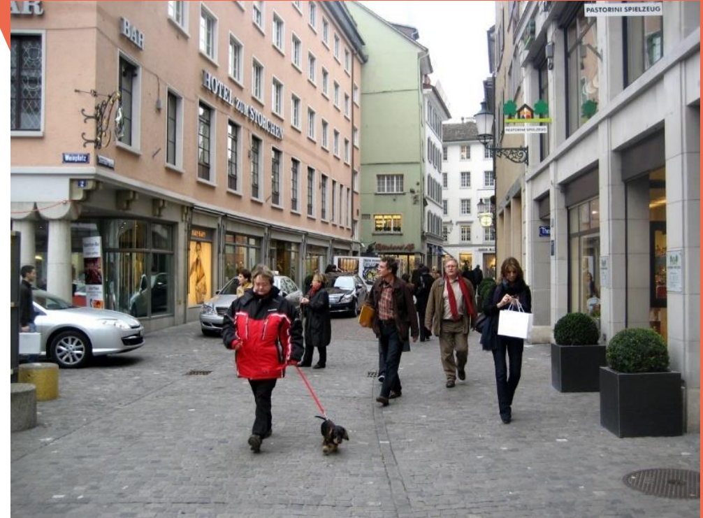
Shared space scheme in Zurich, Switzerland. Note the lack of kerbs or tactile surfaces, making navigation for visually impaired pedestrians difficult (2030 Palette, n.d.).
